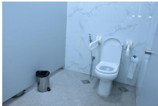
Bathrooms for people with special needs
